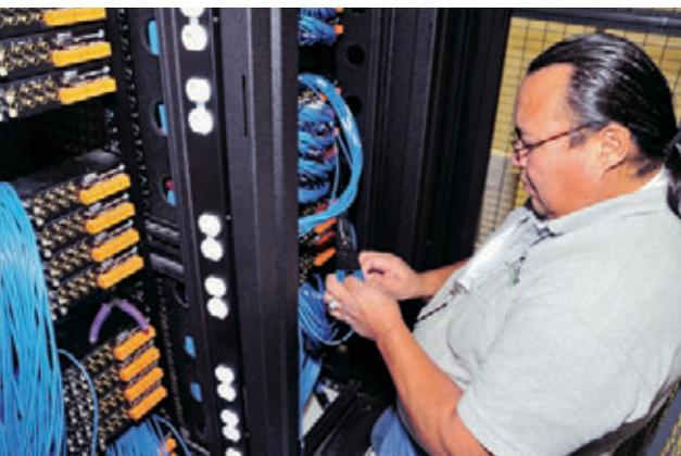
Daryll Mouse of Technical Security Integration (TSI) wires up the paddleboards for Synectics' internal PCI-e 16-channel encoders.
